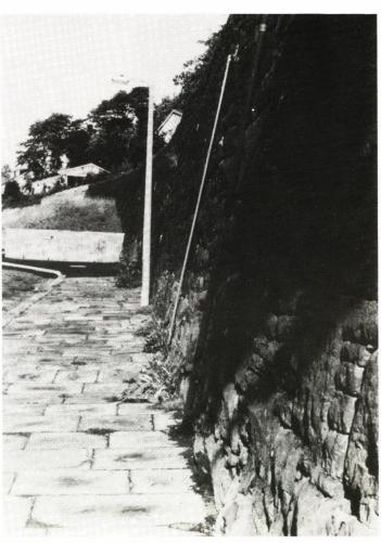
Fig. 2. View showing typical batter of dry-stone walls
