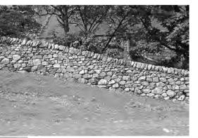
Above wall on slope showing jumpers and levelling. Left similar construction but on the flat. Both Blaen y Nant, Nant Ffrancon. Both © Sean Adcock
