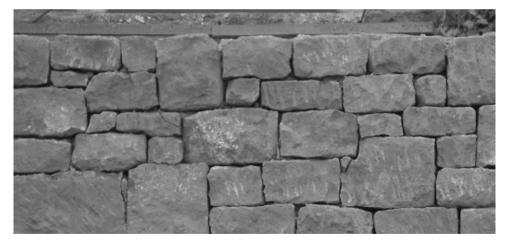
Random Snecked wall, Catesby, Northamptonshire © Sean Adcock This piece of dry face mortar backed retaining wall shows how snecks and jumpers mixed together can create a random wall out of regular stone.
